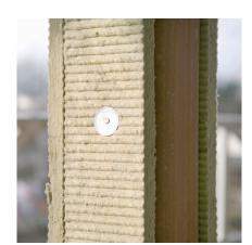
The boards should form a solid corner on the steel profile. No steel shall be visible.
