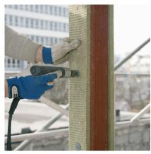
The welding is done by PAROC Pin Welding Device – or equal.
