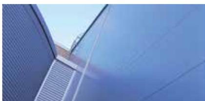
Sandwich panels are fire proof lightweight steel-faced panels with a core material of stone wool. Paroc panels are used for façades, partitions and ceilings in public, commercial and industrial buildings.
